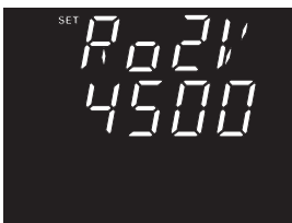
Figure 3-59 RO2/DO2 alarming setpoint setting
